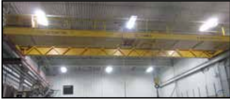
PRO-ACTION 5 TON BRIDGE CRANE
